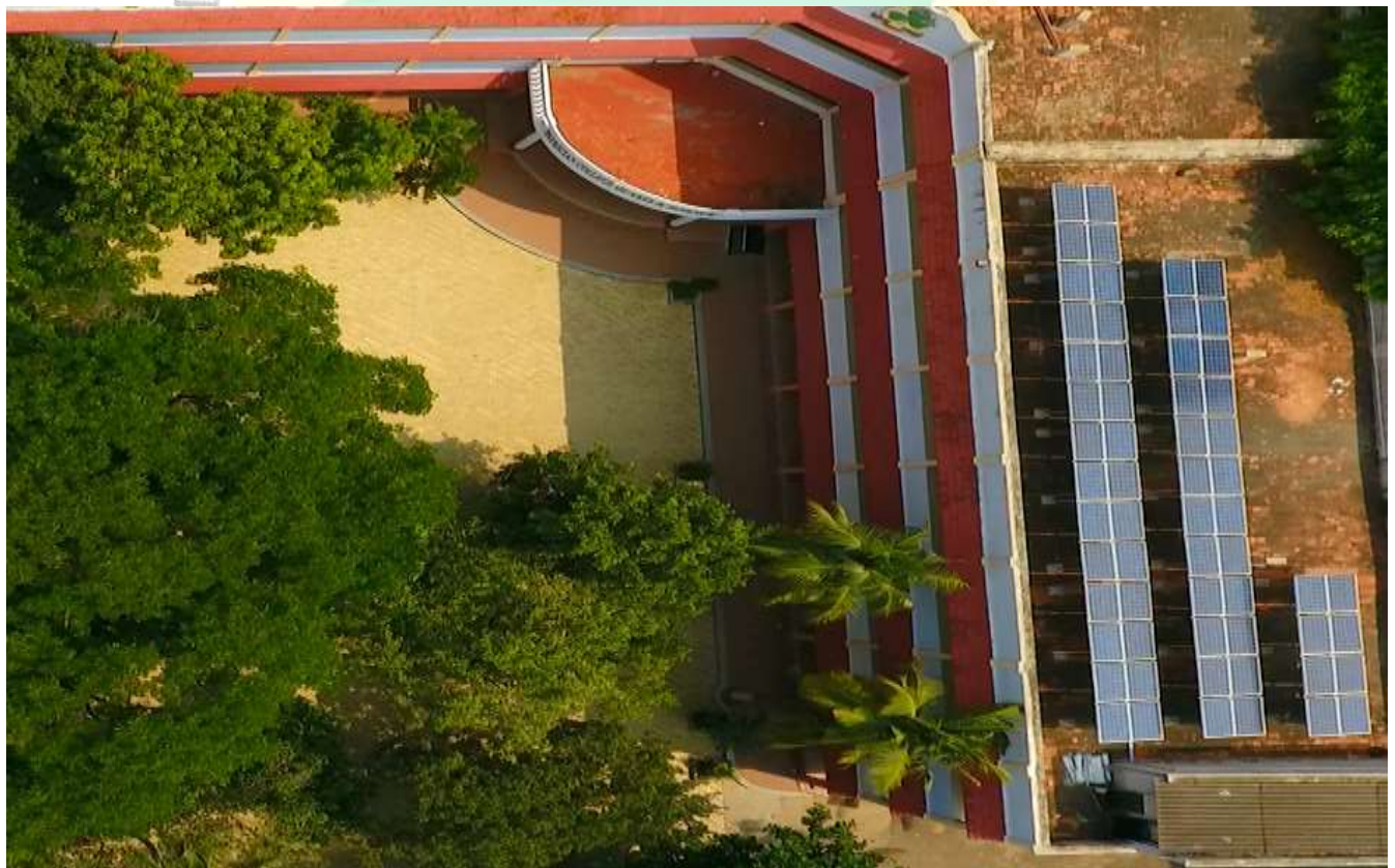
Bird's Eye View – Solar panels
