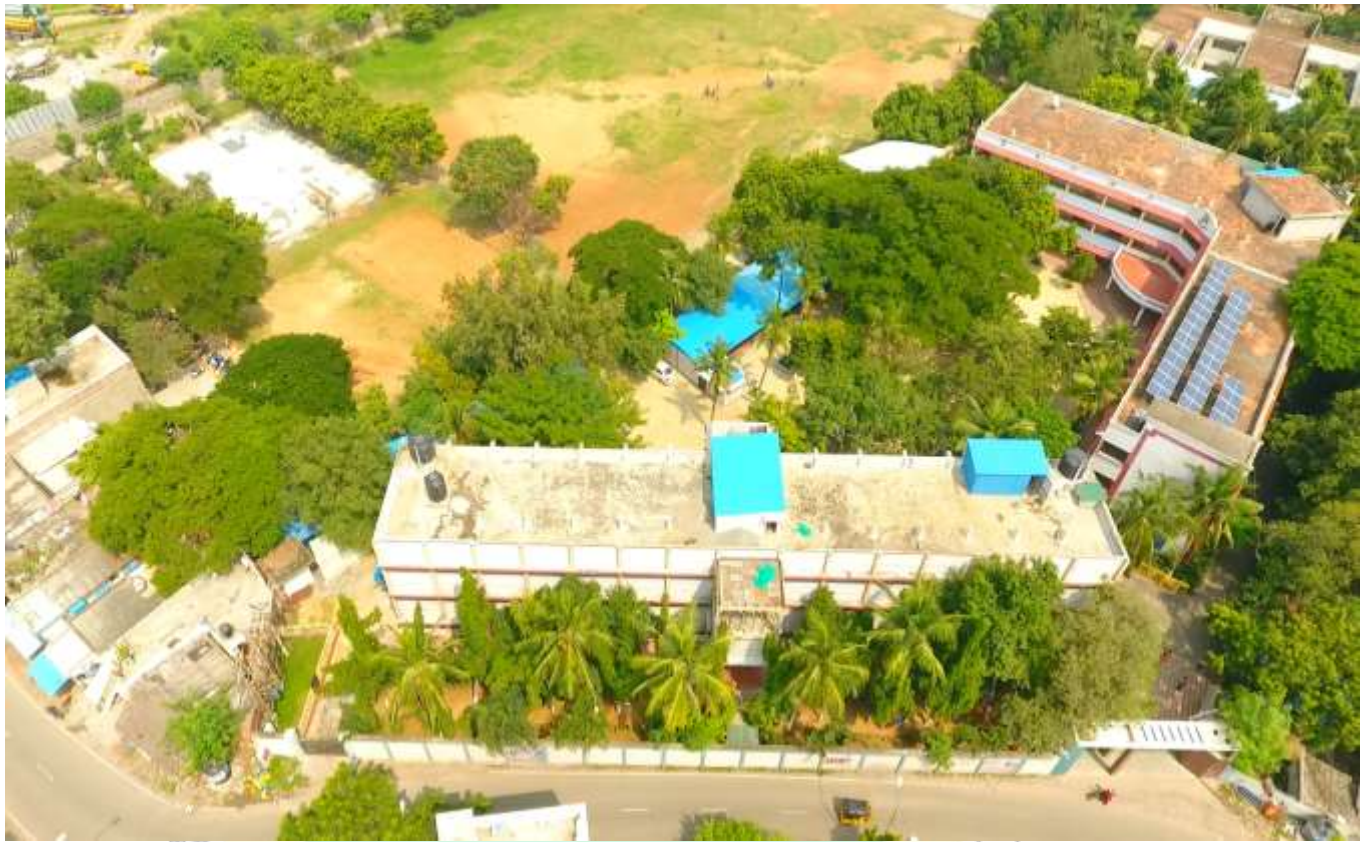
Bird's Eye View – Solar panels
